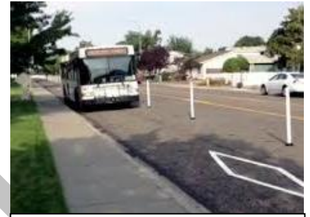
Figure 3C. A separated lane with posts (also known as bollards)
