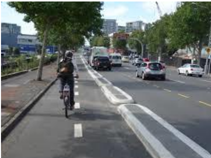
Figure 3A. A separated lane with small concrete barriers.
